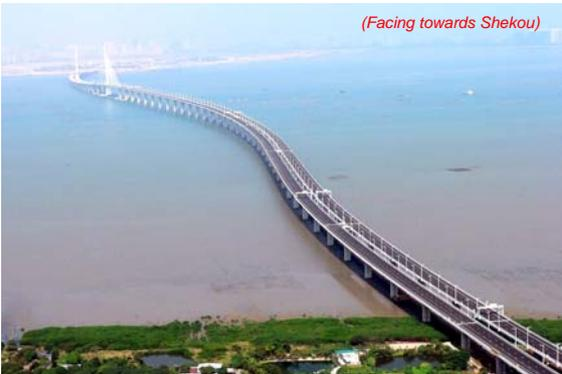
HK-SWC comprises a viaduct section with typical span of 75m in the form of a precast segmental prestressed concrete box girder, a section of viaduct with span of 75m in the form
