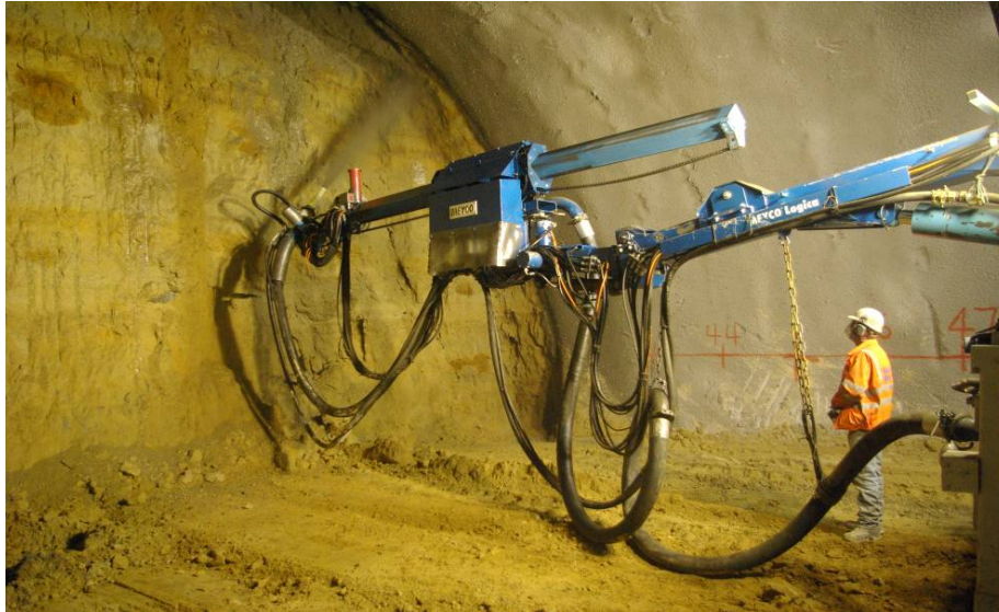
Figure 3 – Primary Lining Application
