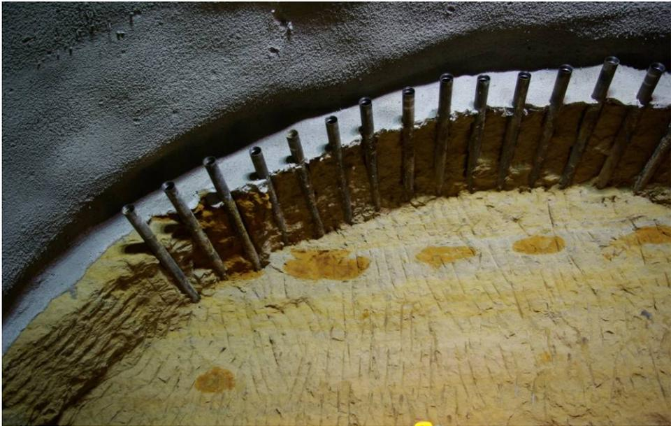
Figure 5 –Typical Canopy Tube Installation
