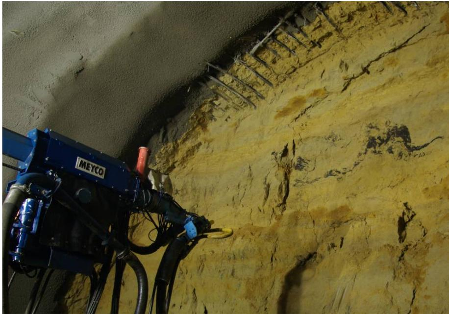
Figure 4 –Typical Spile Installation
