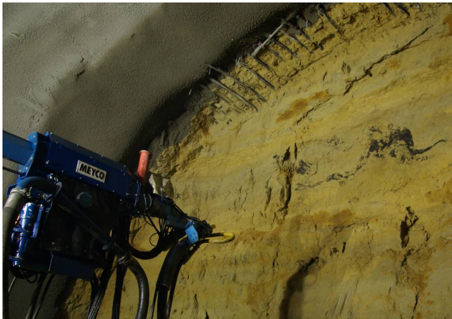
Figure 4 –Typical Spile Installation
