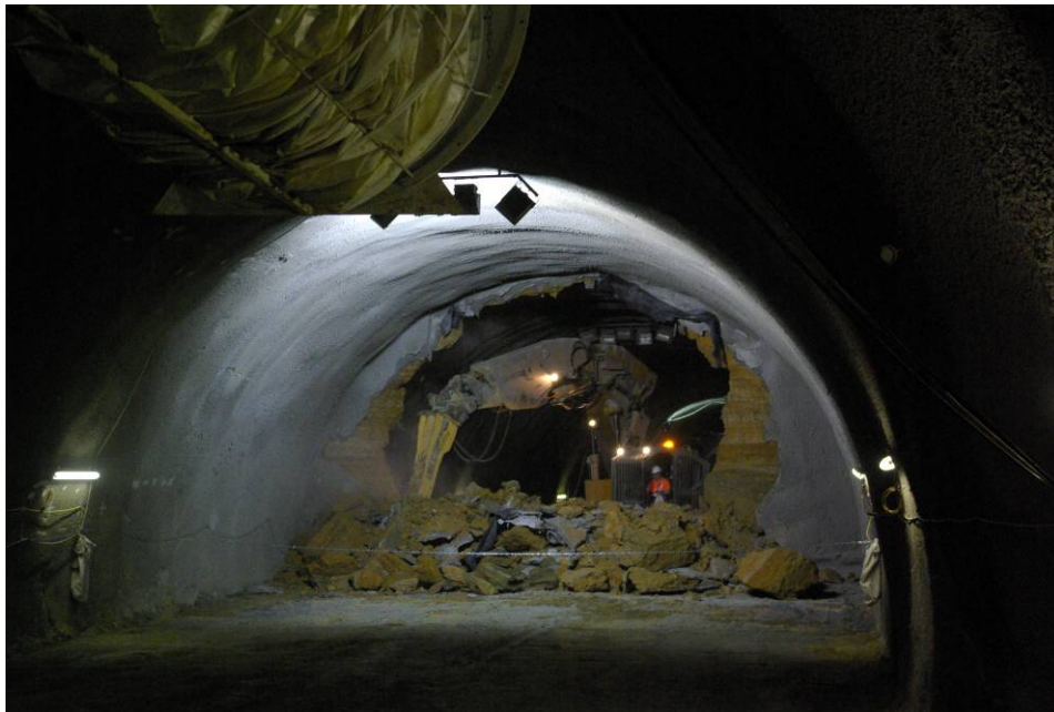
Figure 6 – Tunnel Breakthrough, February 2009
