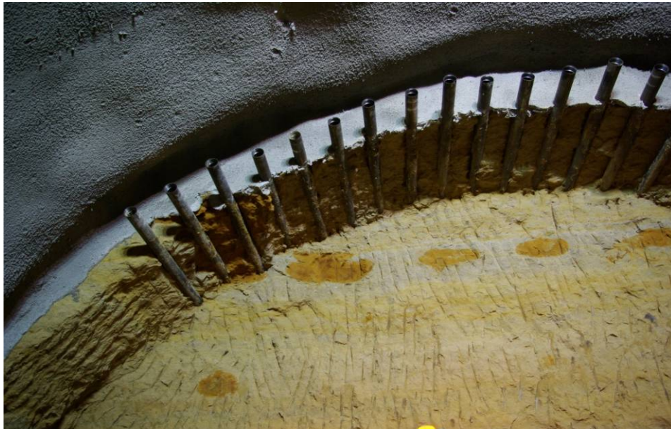
Figure 5 –Typical Canopy Tube Installation
