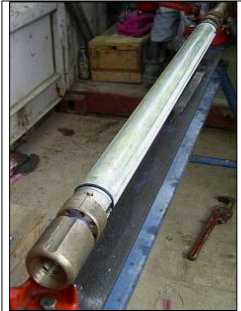
Figure 5 – Directional Drilling in Hong Kong.
