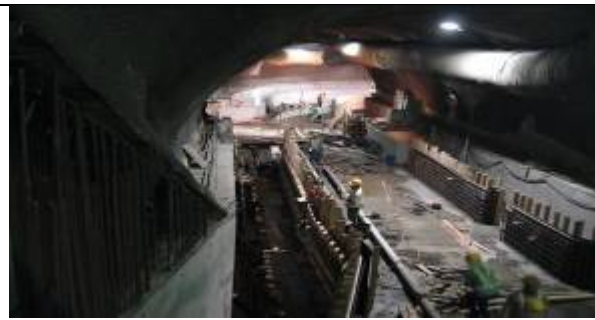
Figure 2a – Saltwater reservoir cavern at Hong Kong University, Hong Kong, 2008-2010.
