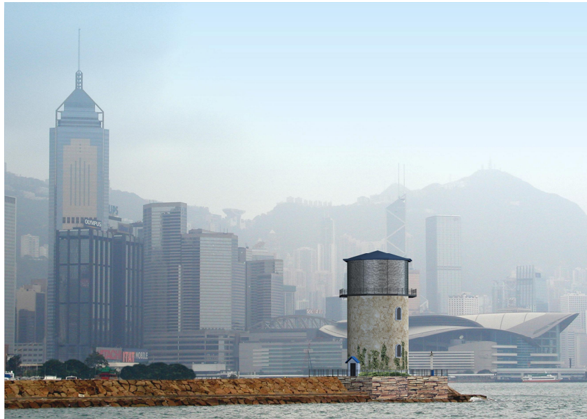
Figure 3.2.2: Vent Shaft Located in the Eastern Breakwater of the CBTS (Design of vent shaft shown is tentative only)
